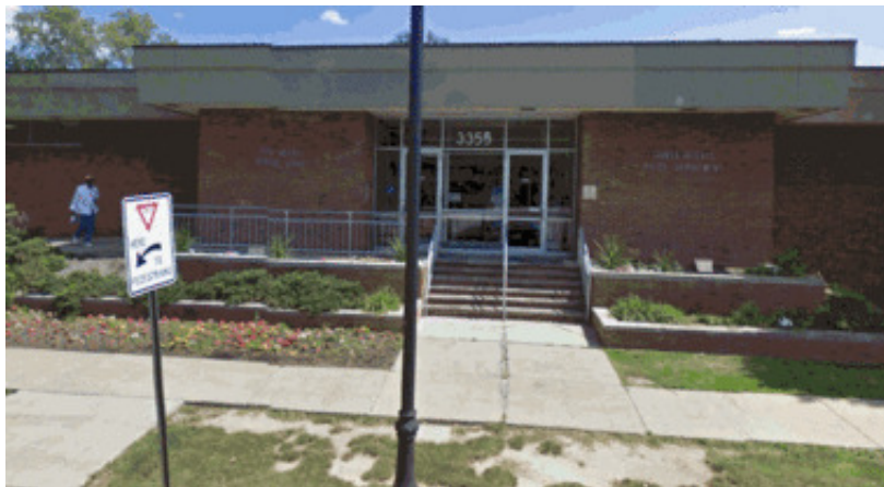
Shaker Heights Municipal Court
